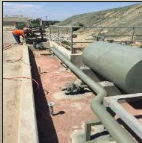
Priming of piping and tanks
