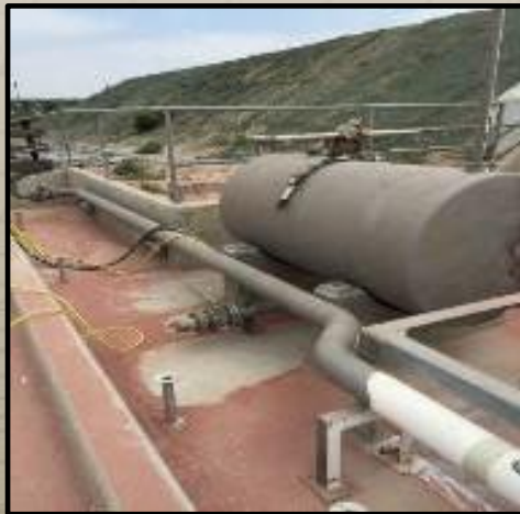
Sandblasted to bare metal
